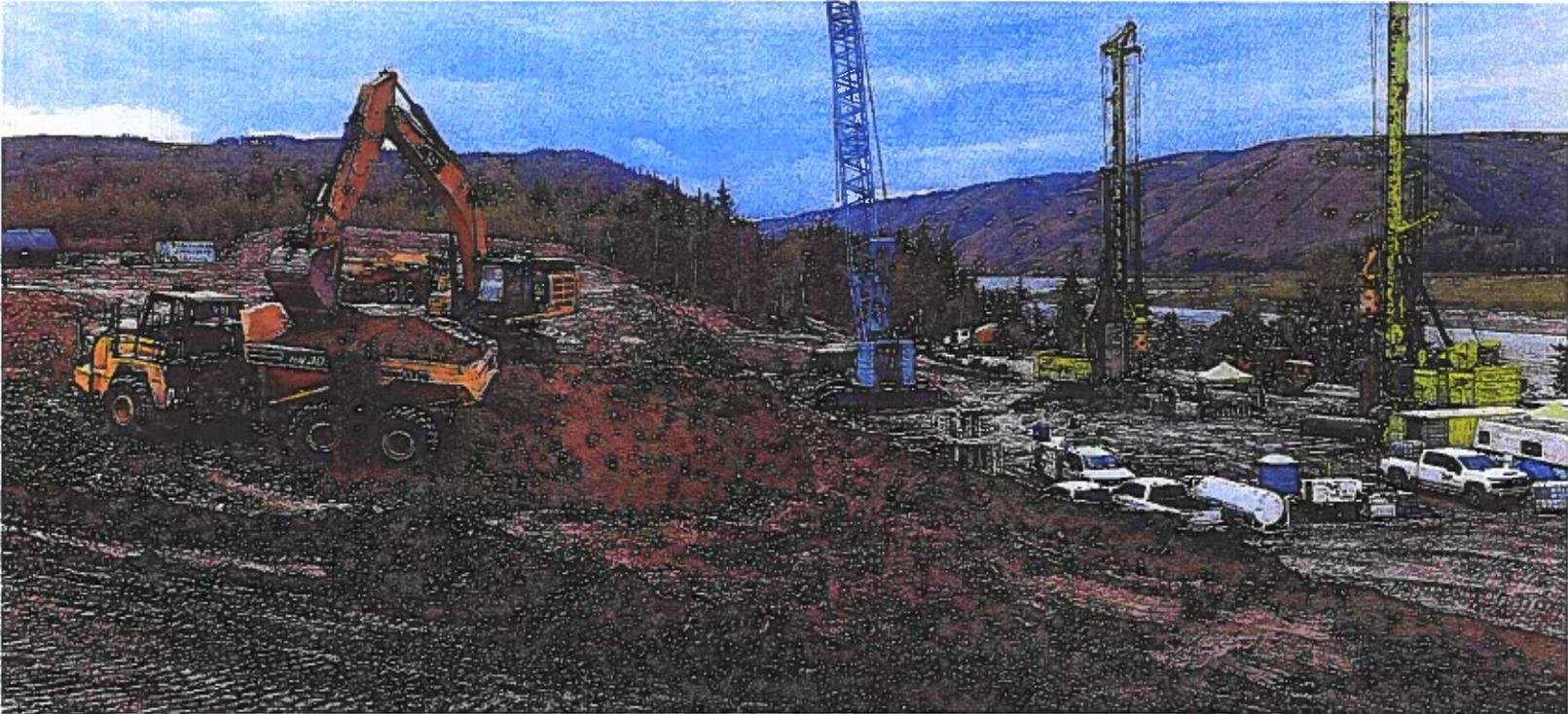
3. Overhead View for Installation of Concrete Guide Wall for Secant Pile Wall Shoring System for Raw Water Wet Well
