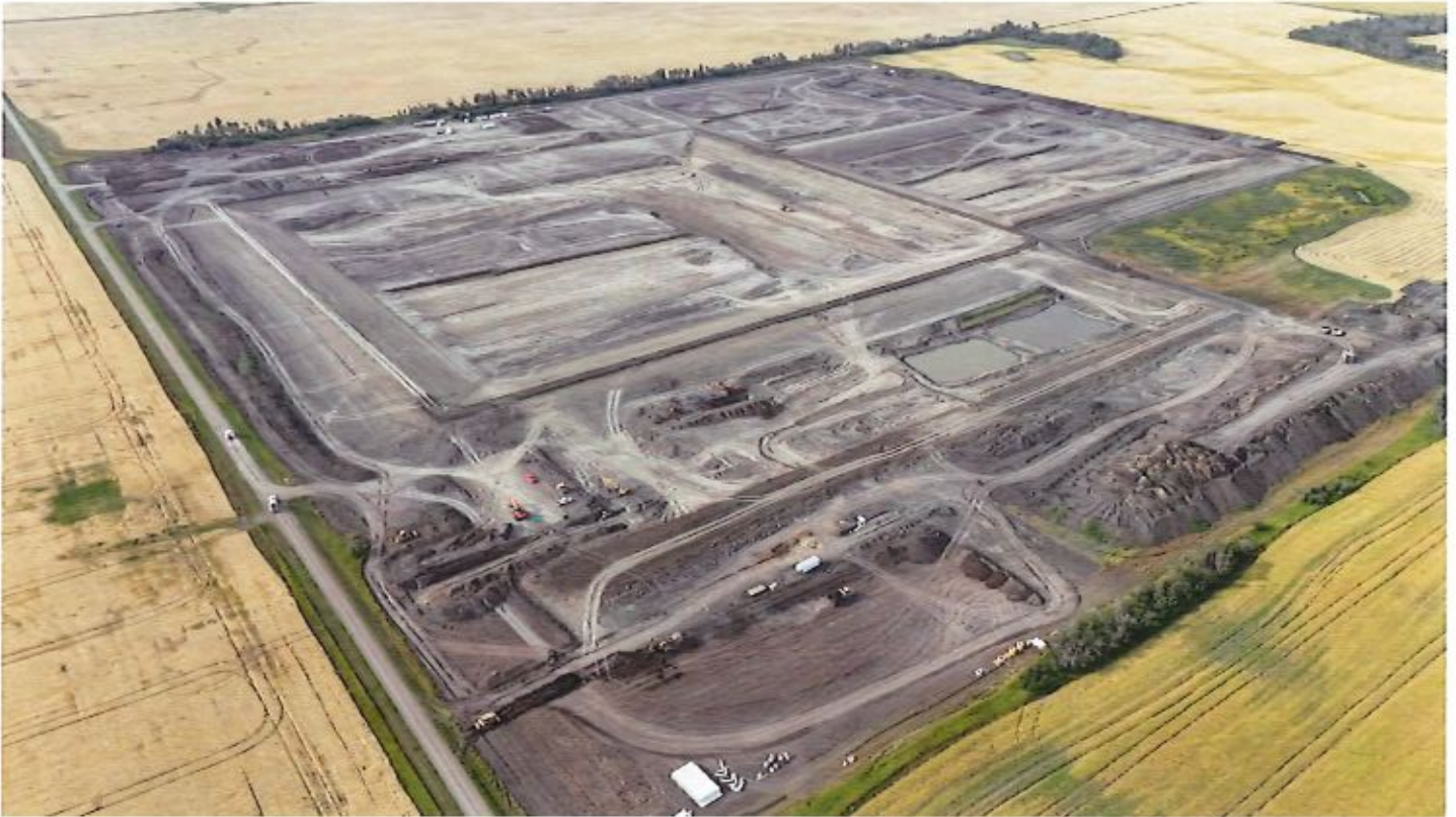
7. Phase 3 Contract 1A Raw Water Reservoirs – View Looking Southwest
