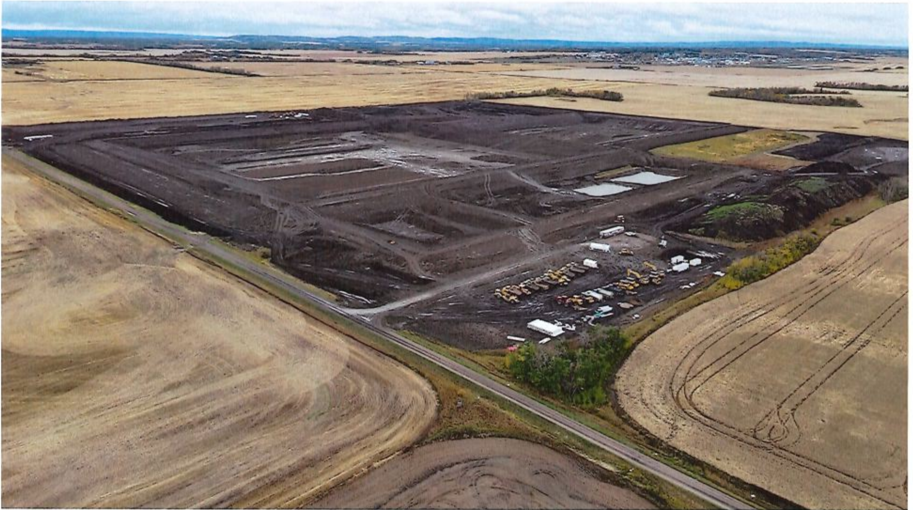
13. Phase 3 Contract 1A Raw Water Reservoirs – View Looking Southwest
